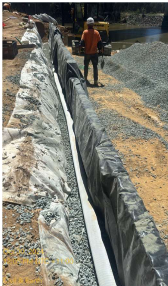
Figure 5 – Agi-drain Installation
