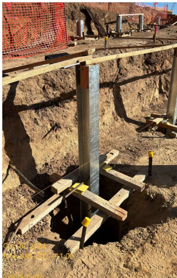
Figure 4 – 150 UC Installation
