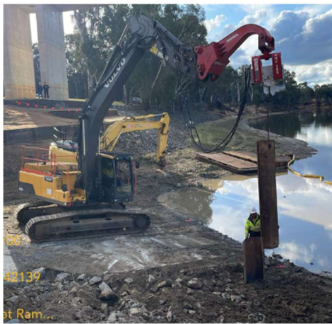
Figure 8 – Sheet Pile Installation
